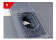
Fix vent by nailing through centre nail holes. Place the adjacent slates around the Slate Vent accordingly.
