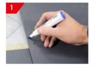
Mark the position for the Slate Vent by drawing a box with a cross as shown above.
