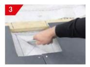
Carefully cut the underlay diagonally on the marked cross and peel back the underlay to the surrounding batten and under the slates for the sides.
