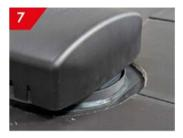
The two slates on the course above will need to be cut around the upstand of the slate vent. The slates should not touch the upstand; a 10mm gap should be maintained.
