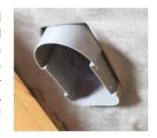
If the vent tile is being used for roofspace ventilation only, the spigot on the back of the vent tile should be left open as shown'
