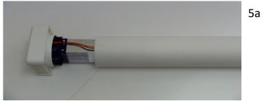
See Fig 5a, 5b & 5c Next slide the outer tube OVER THE INNER TUBE and mark off the length as you need to cut this to the same length as the inner tube. 4.
